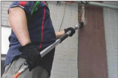
Corrosion removal for inaccessible area
